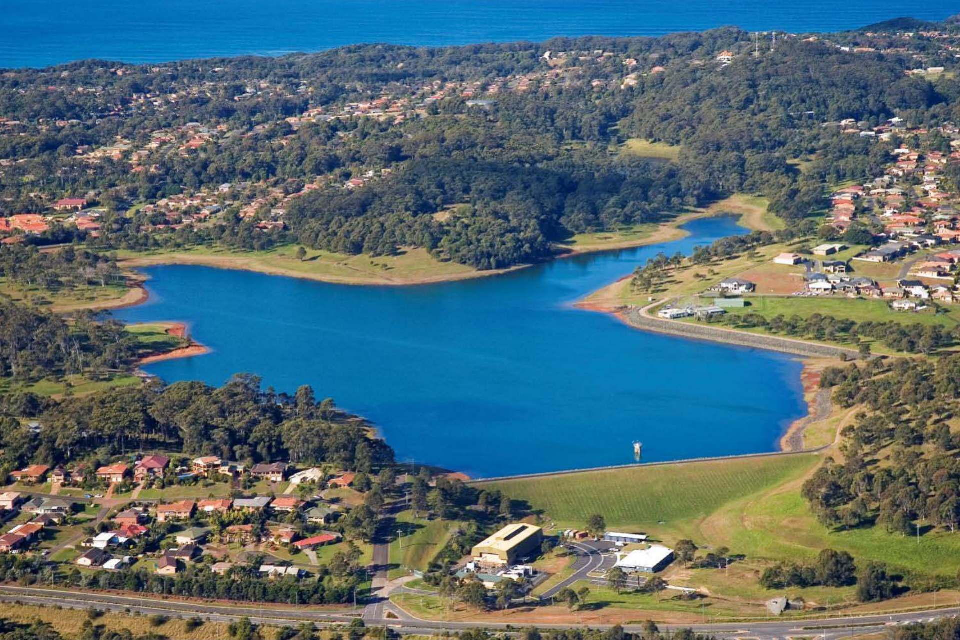
Port Macquarie Off-Creek Storage Dam – 2,500ML
