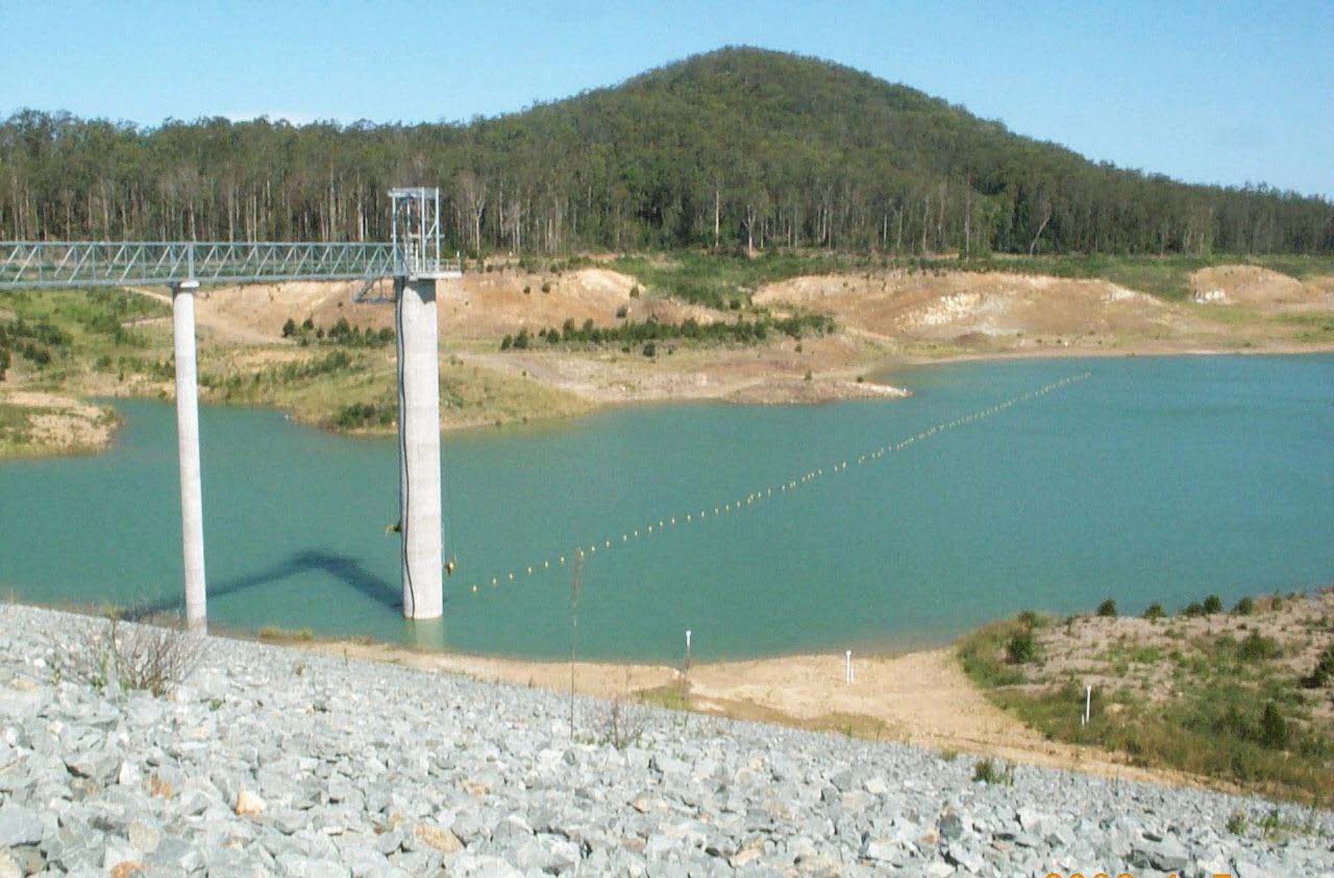
Submerged Aeration System & Mixer Units on Intake Tower
