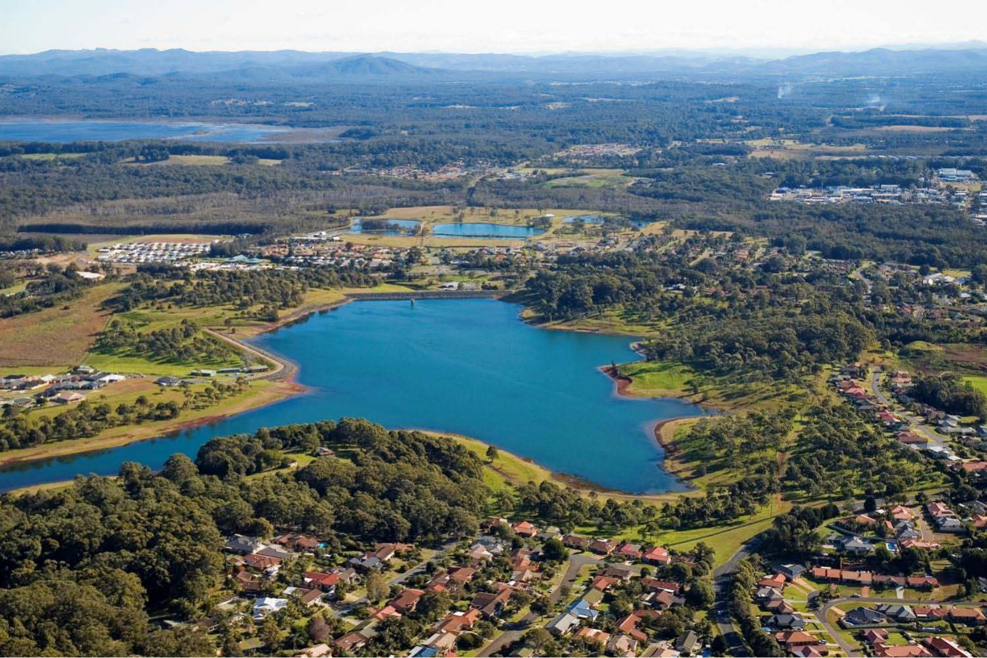
Downstream Development of Port Macquarie Dam
