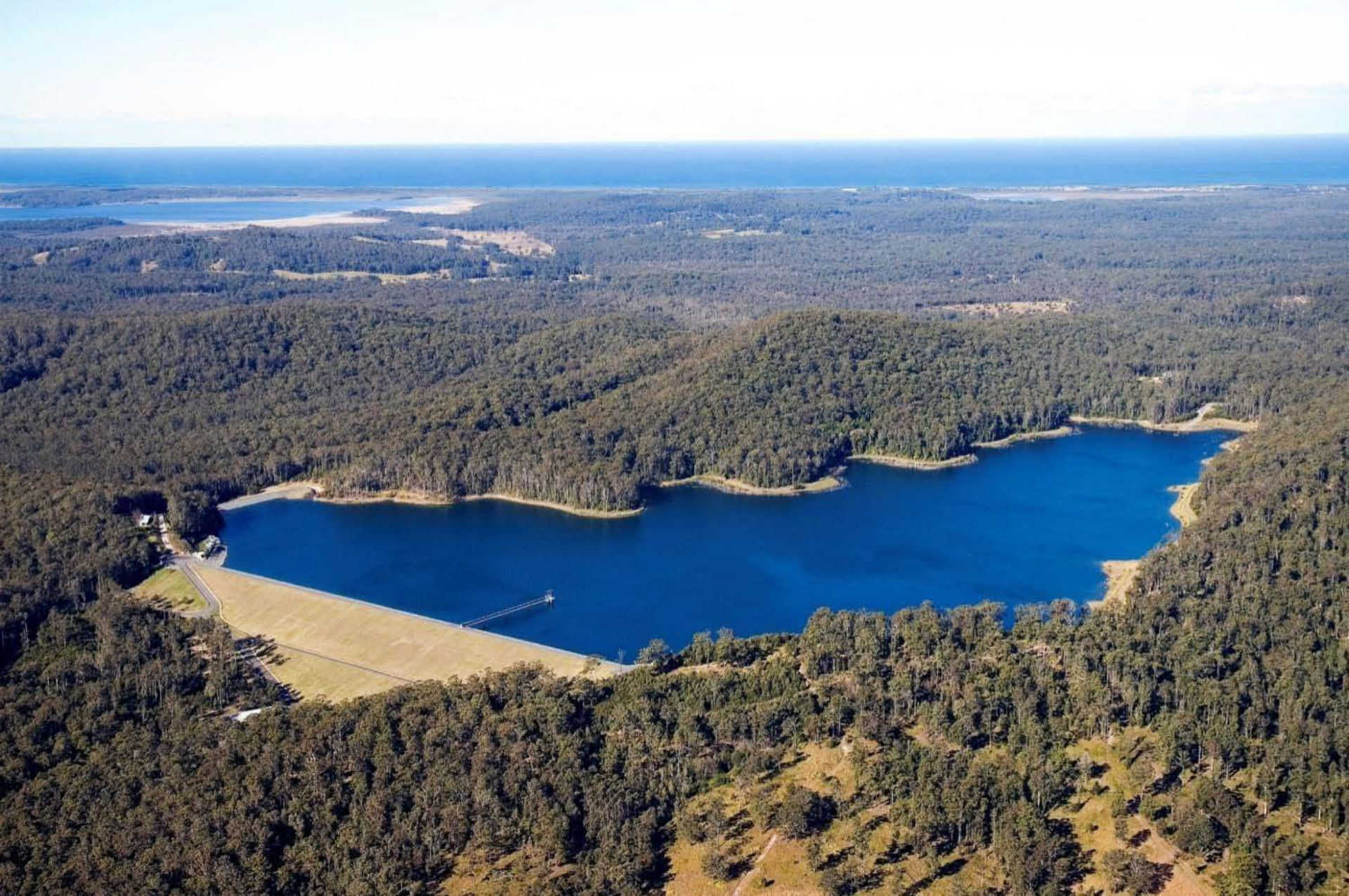
10,000 ML Cowarra Off-Creek Storage Dam
