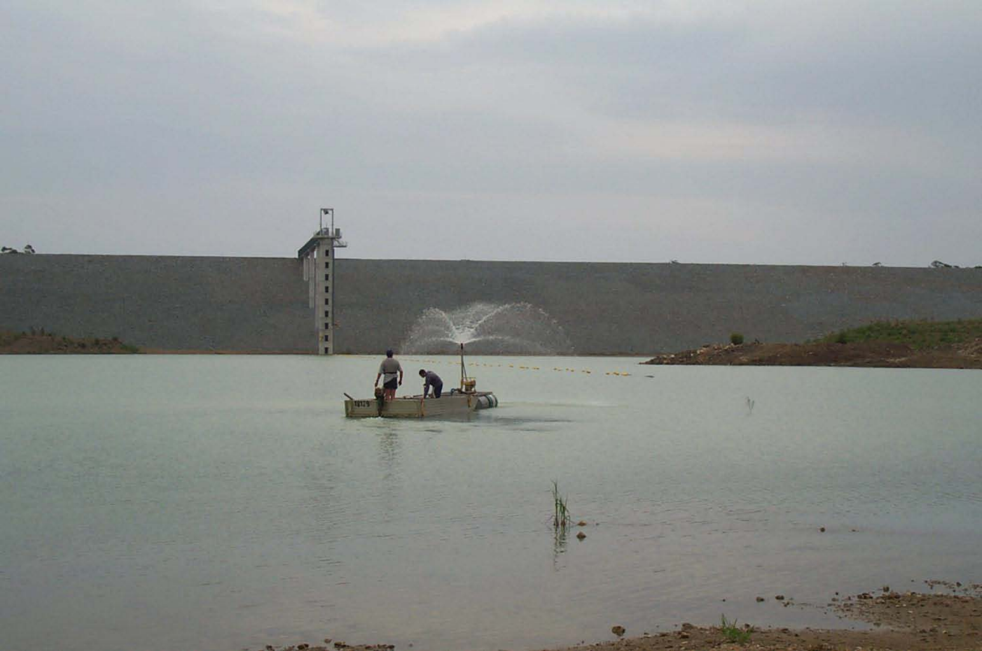
Gypsum Application Using Spray Unit
